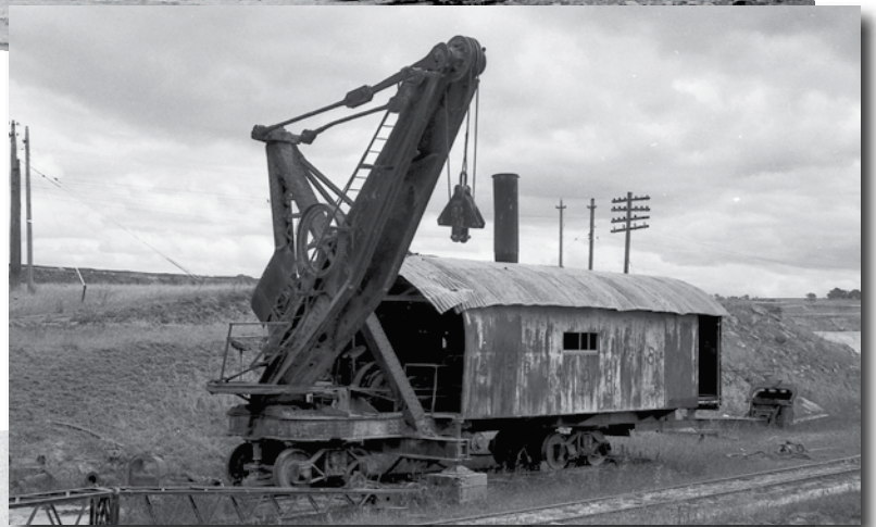
Above: Number 6 (at right) a four-wheel steam railway grab crane, built by Ruston & Hornsby, has 'tracked' Ruston number 3 for company in its retirement. 12 January 1965. Photo: Richard Horne
