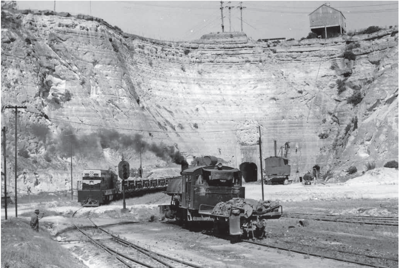
Above: D1 and number 4 meet up inside the quarry on 27 January 1966. Photo: Richard Warren, collection Richard Horne
