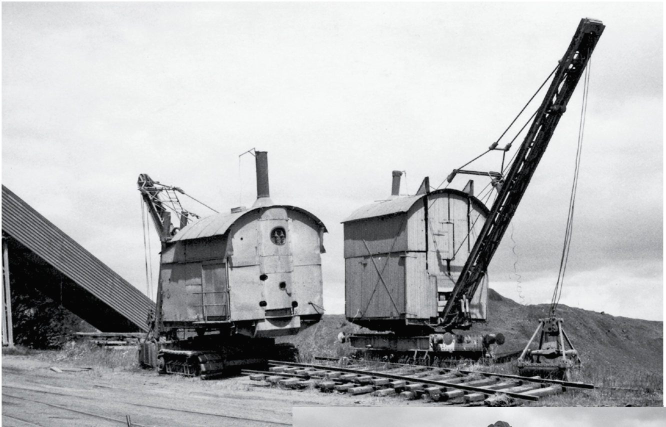
Above: Number 6 (at right) a four-wheel steam railway grab crane, built by Ruston & Hornsby, has 'tracked' Ruston number 3 for company in its retirement. 12 January 1965. Photo: Richard Horne
