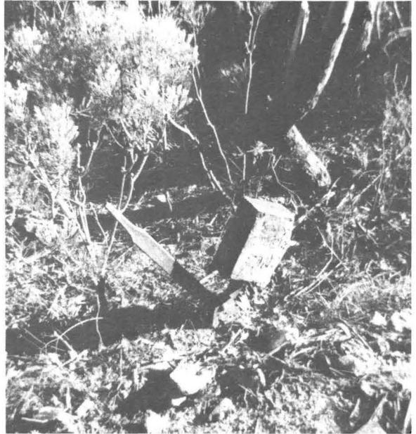
Lever as used on Mt. Victoria Incline. Inscribed on concrete portion of lever is "NL 1926". There were three (3) of these levers on the incline. When this photo was taken, this lever near the incline summit was still "in situ". Since being taken the lever has since been removed, by no doubt vandals. Photo taken on Sunday 27th April, 1975. The two (2) other levers were located and are still in their original positions about halfway on the incline.
