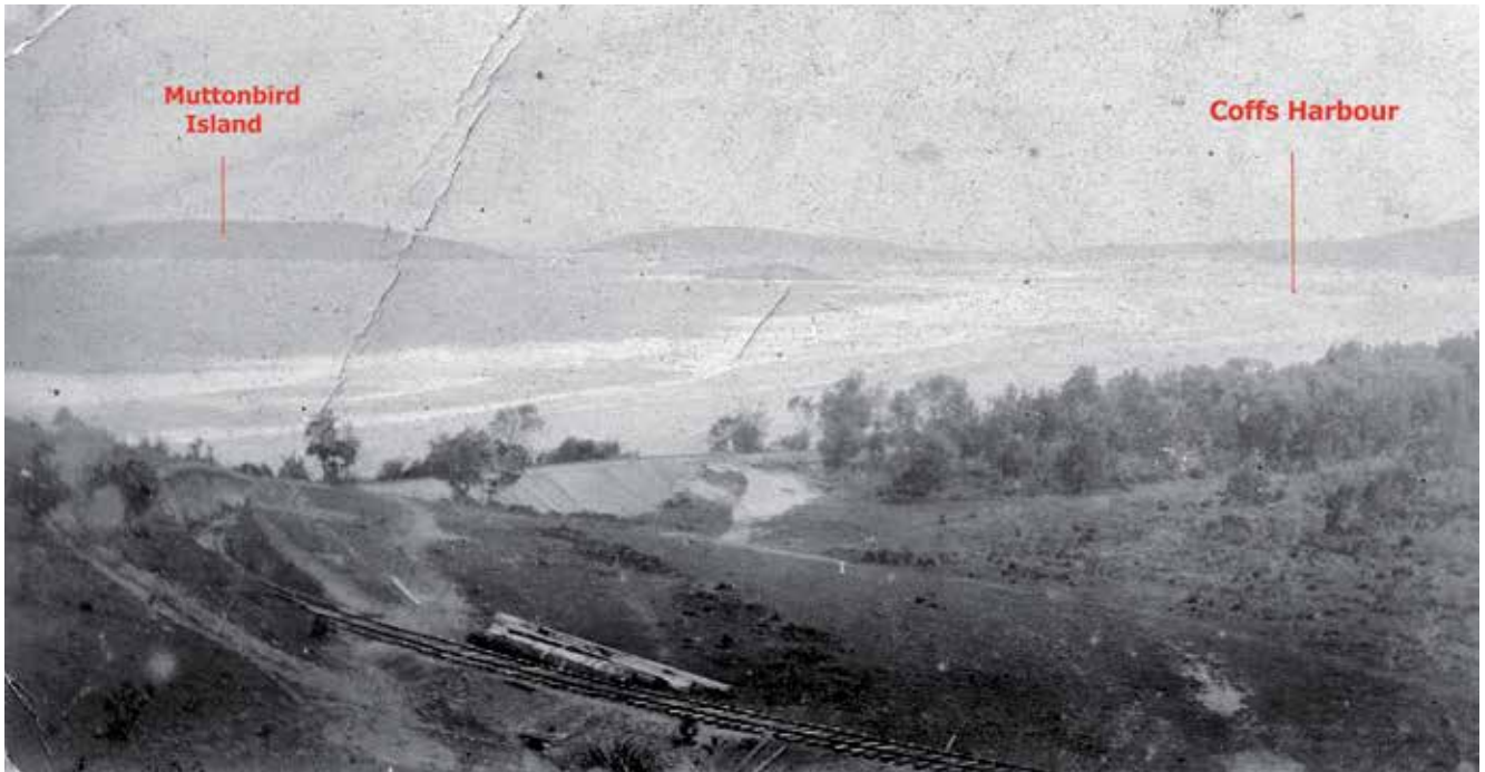
The BATCo's timber tramway at Macauleys Headland, Coffs Harbor c1910. The line climbed up from the coastal plain on the right by means of a substantial embankment and a deep cutting. The embankment is long gone but the cutting could still be found (in 2012) amidst trees on the southern face of Macauleys Headland Reserve. Photo: Coffs Harbour Regional Museum
