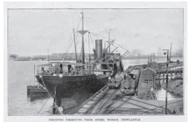
SHIPPING PRODUCTS FROM STEEL WORKS, NEWCASTLE
