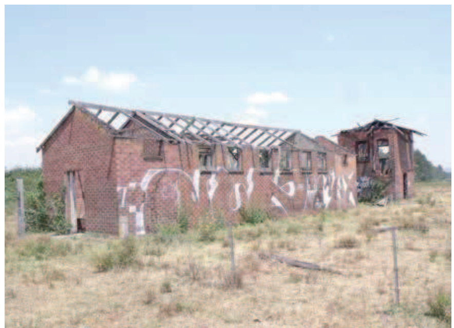
The remains of the bathhouse and control cabin at Hexham, located not far from the now-demolished engine shed, 7 October 2012. Photo: Brad Peadon
