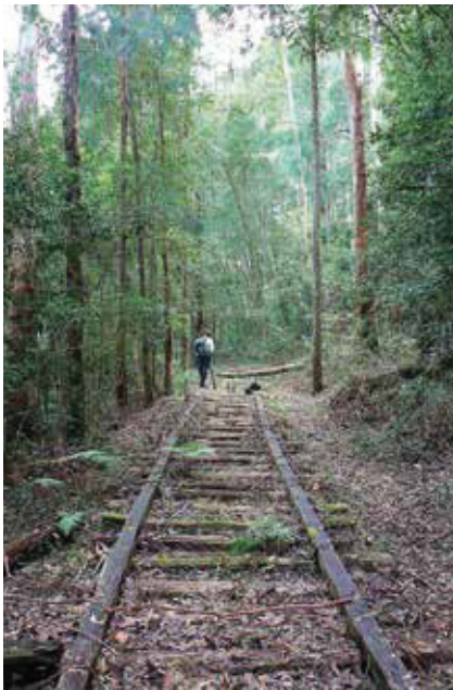
The section of replica wooden railed tramway, built by the Kendall Historical Society.
