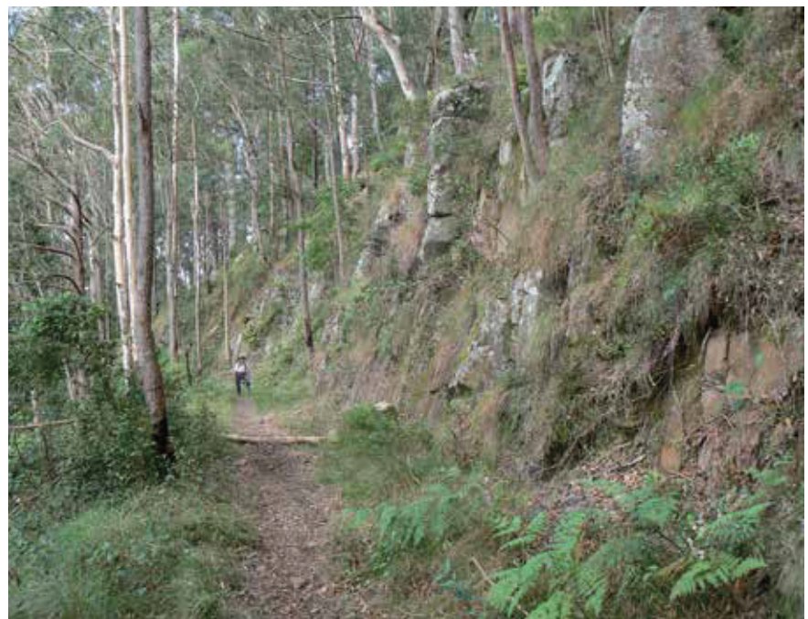
An impressive tramway ledge on the 1924 Winns Hill line of the Simsville timber tramway, about one kilometre short of the former terminus.
