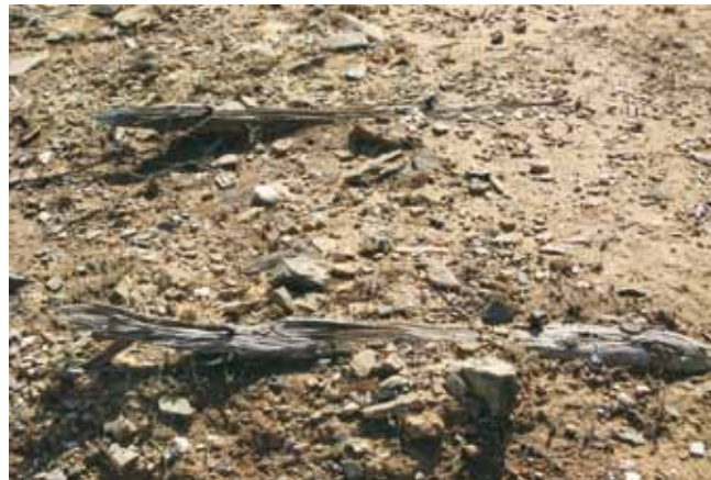
2ft gauge sleepers in Quarry K with spikes still in place. Photo: Chris Wurr
