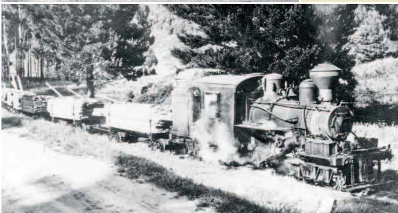
The Harman geared locomotive on a 5ft 3in gauge flat wagon ready for transport to Moe. Photo: LRRSA Archives □ Climax locomotive No.1694 at Tyers Junction in the 1930s. Photo: Forests Commission Victoria □ No.1694 leaving Tyers Junction with a load of sawn timber bound for Collins Siding, in the late 1940s. This shows the locomotive with the new welded smokebox which was made by the FCV. Photo: AP Wymond, courtesy Mike McCarthy
