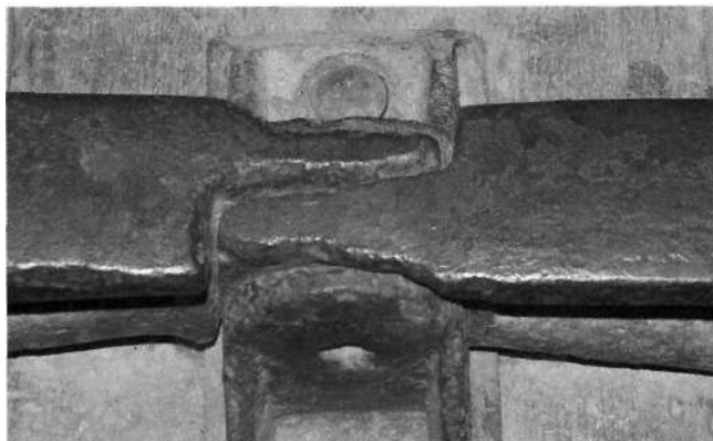
Scarfed ends of fish-bellied rails in an iron chair displayed at the Science Museum, in London. Photo: Bob Cook
