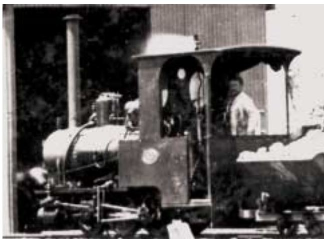
No.3444 shown working at the Lake George mine.
